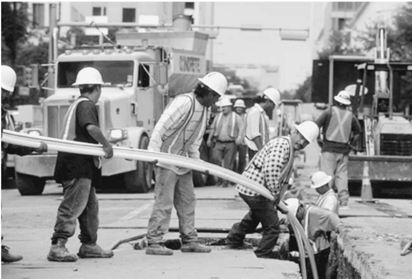
Workers laying fiber-optic cable in downtown Austin, Texas. Fiber-optic technology has made it possible to transfer streams of data virtually error-free and at rates that far exceed those of previous technologies. (Bob Daemmrich/The Image Works)
