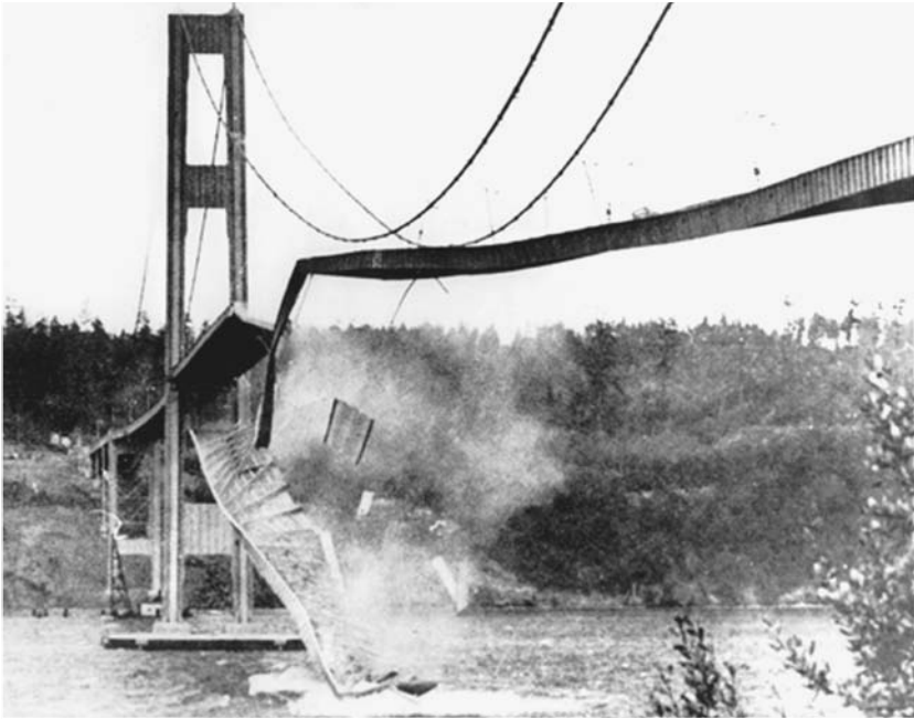
The Tacoma Narrows Bridge, November 7, 1940, a famous example of the phenomenon of resonance. The wind caused the bridge to begin to oscillate. Continued wind caused the amplitude of the oscillations to slowly increase until they tore the bridge apart. [Topham/The Image Works]
